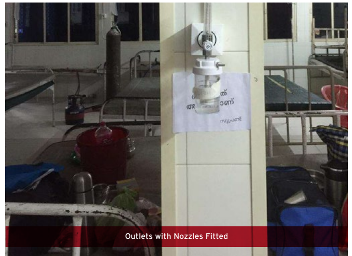
Wards with Oxygen Pipes Installed
